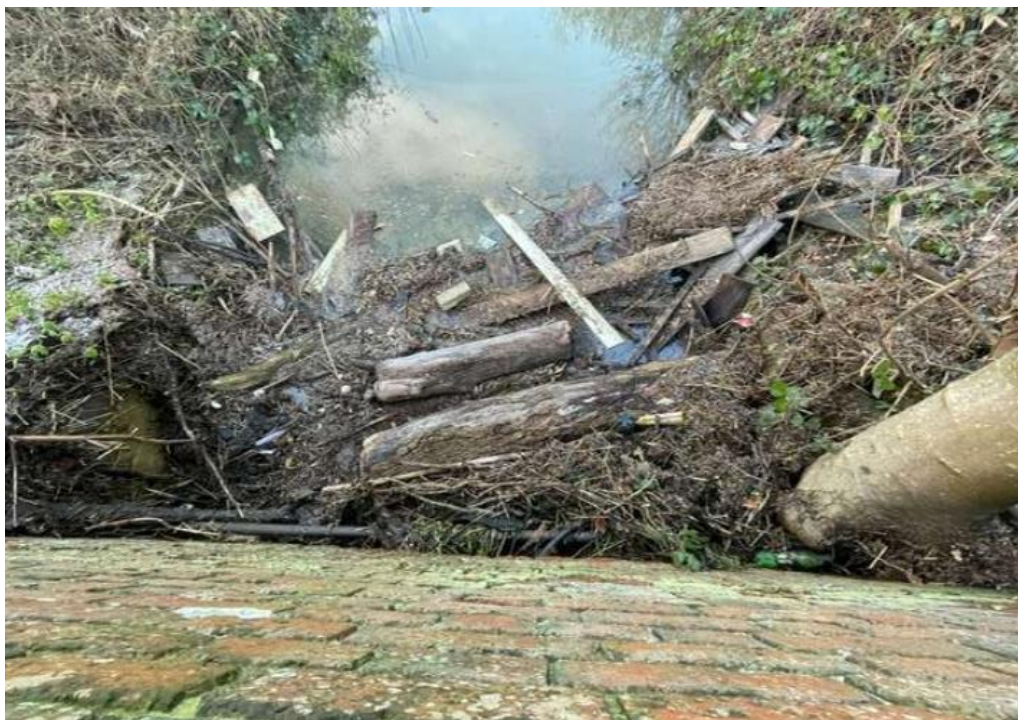
Blockage of culvert by woody debris, eastern end of Hills Meadow, Lower Caversham
